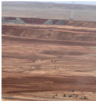
The floor of unlined Tailings Cell2 at OT likely to result in mine tailing leakage and water contamination. Image: July 2023
