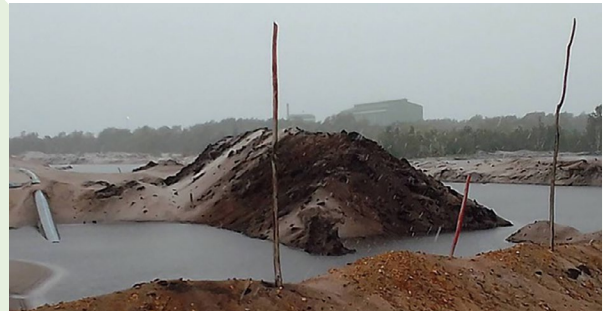
Mine environs after uncontrolled water release, March 2022
