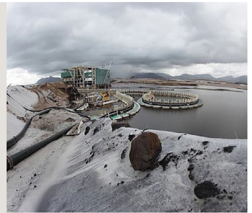
QMM's mine basin and tailings dam
